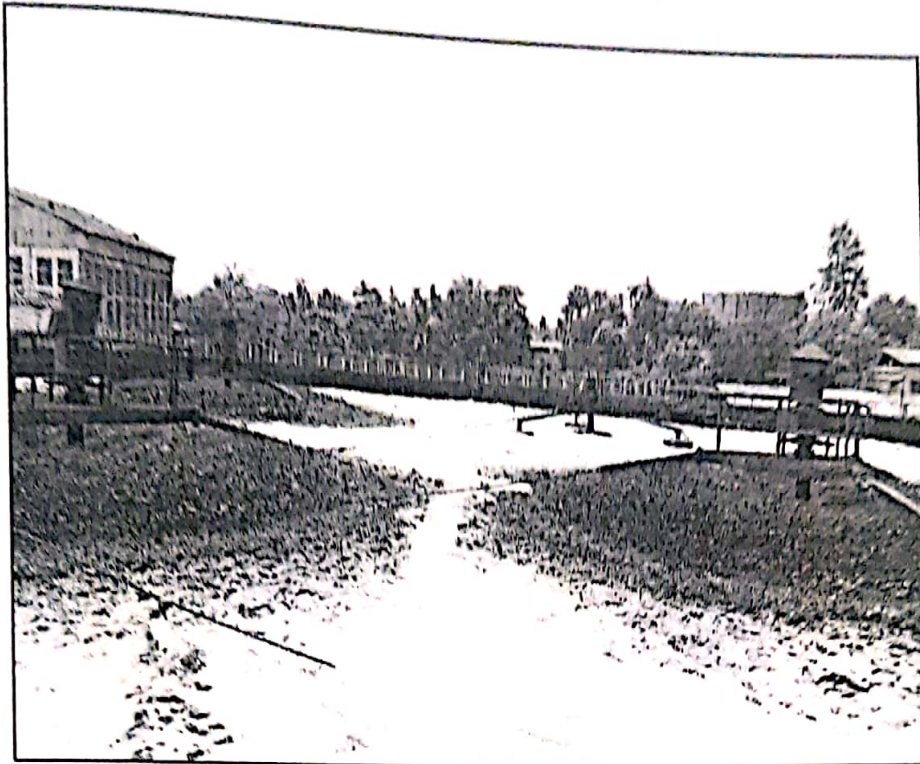
Photo : Aeration Tank
