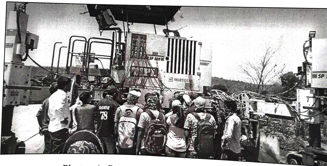
Photo : At Pavement Quality Concrete Machine
