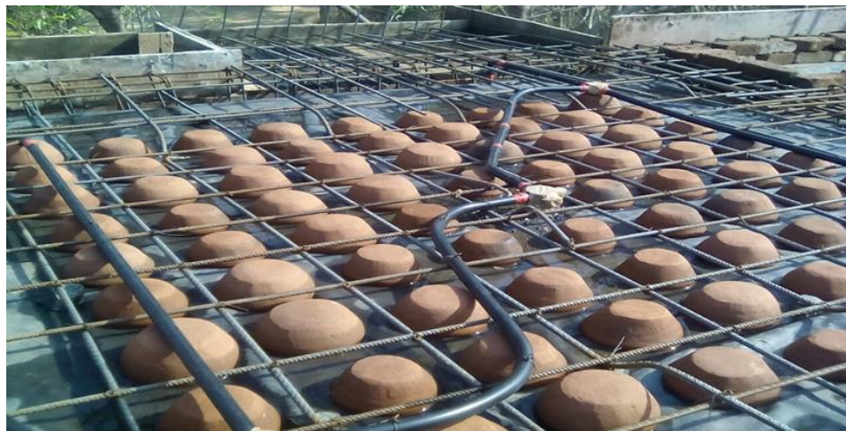
Figure 6. Roofing with Filler Slab
