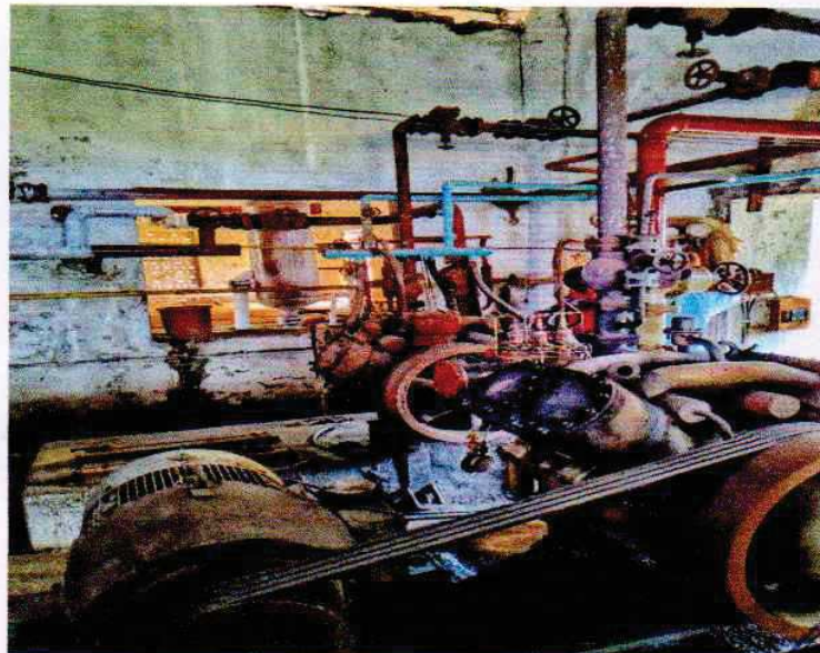
Fig. Compressor used in ICE plant
